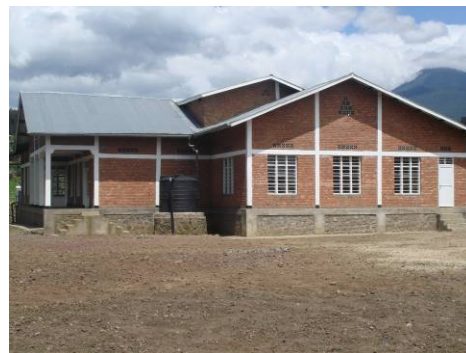
New seed potato storage facility
