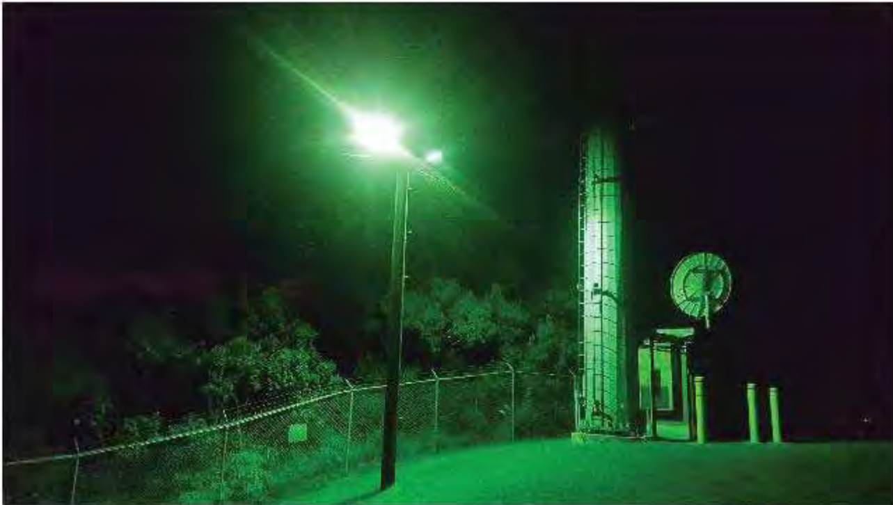
Perimeter Light_C: One green bulb, with full shielding (photo taken after the light was realigned in a downward position).
