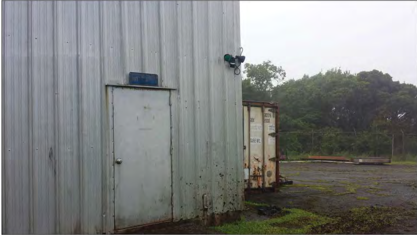
Building 5_Flood Light 2: Two green bulbs, both with shielding and motion detection.
