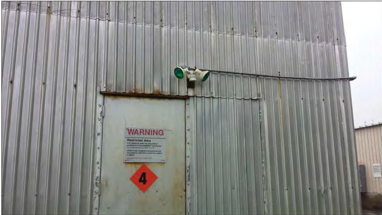
Building 1_Flood Light 2: Two green bulbs with motion detection (close-up).
