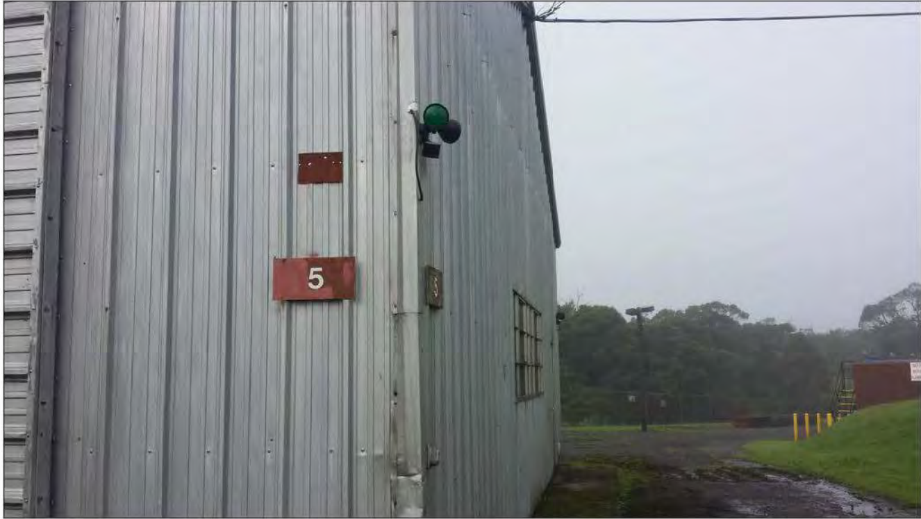
Building 5_Flood Light 1: Two green bulbs both with shielding and motion detection.
