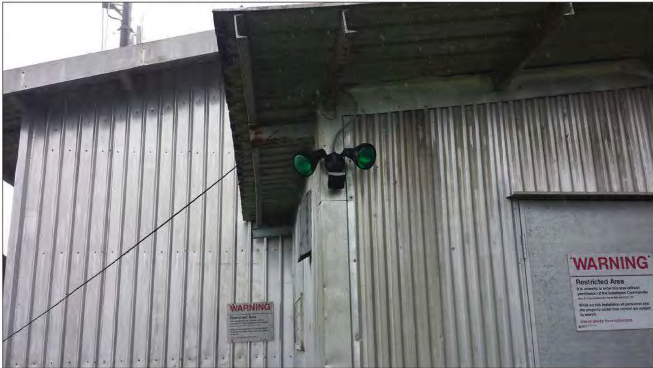
Building 1_Flood Light 1: Two green bulbs with motion detection (close up).
