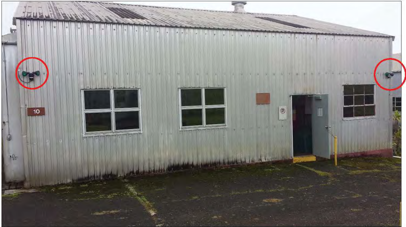
Building 10_Flood Lights 1 and 2: Two green bulbs each, both with shielding and motion detection.
