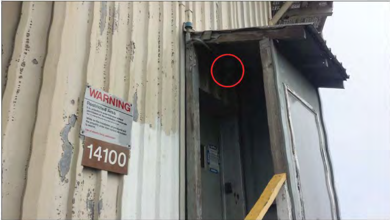
RadarTower_Entryway Light 1: One green bulb with no shielding or motion detection (however the doorway is well blocked by three walls).
