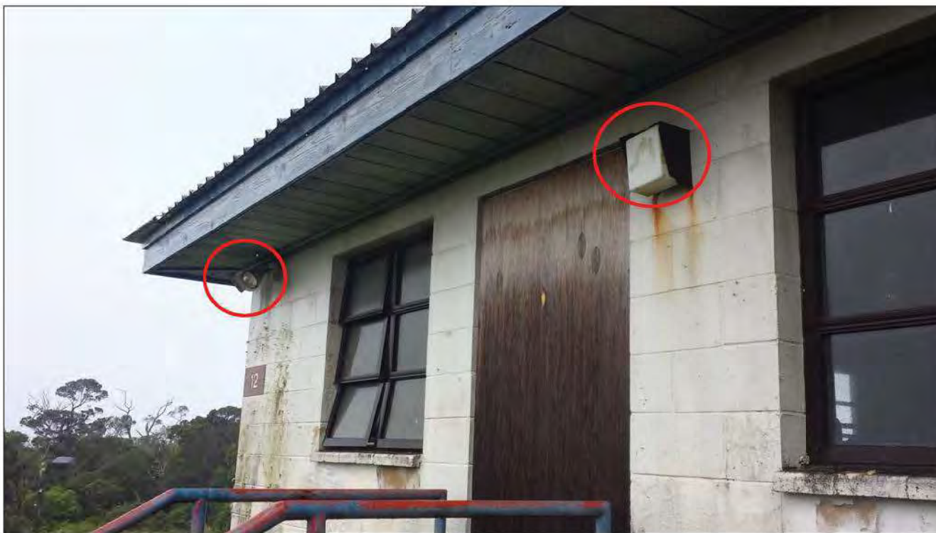
Building 12_Flood Light 2 and Entryway Light 1: Three white bulbs each with shielding and no motion detection (building appears to no longer be in use).
