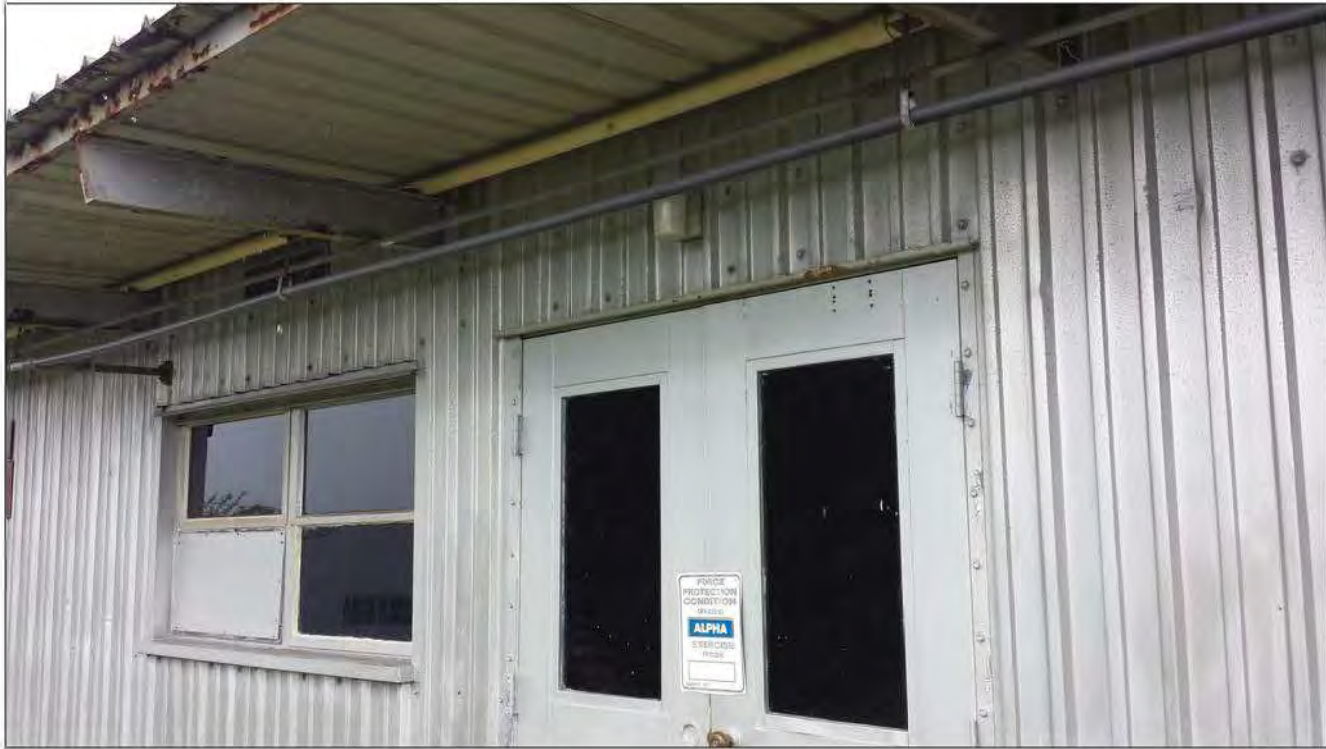
Building 1_Entryway Light 2: One white bulb, no shielding and no motion detection (close-up), 1 st floor, southeast – facing.
