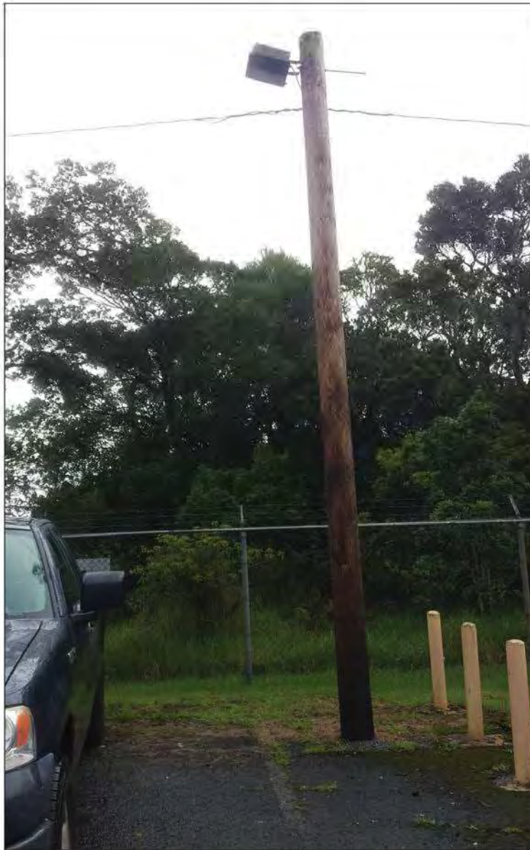
Perimeter Light_B1: One green bulb, with full shielding (light is currently not functioning).
