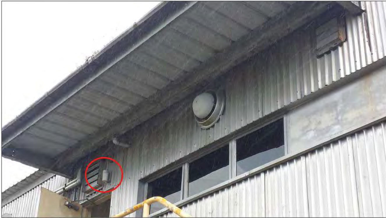
Building 1_Entryway Light 1: One white bulb, with no shielding and no motion detection (close-up), 2 nd floor.
