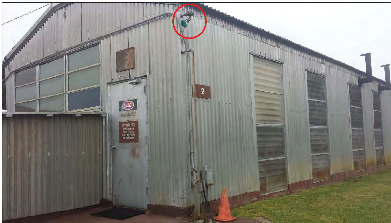
Building 2_Flood Light 1: One green bulb with no shielding or motion detection.
