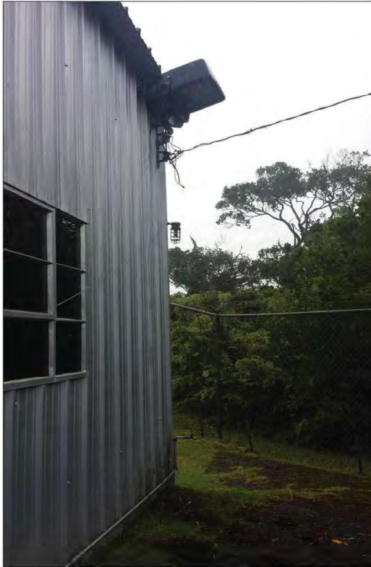
Perimeter Light_O: One green bulb, with full shielding, mounted on the southwest corner of building 5.
