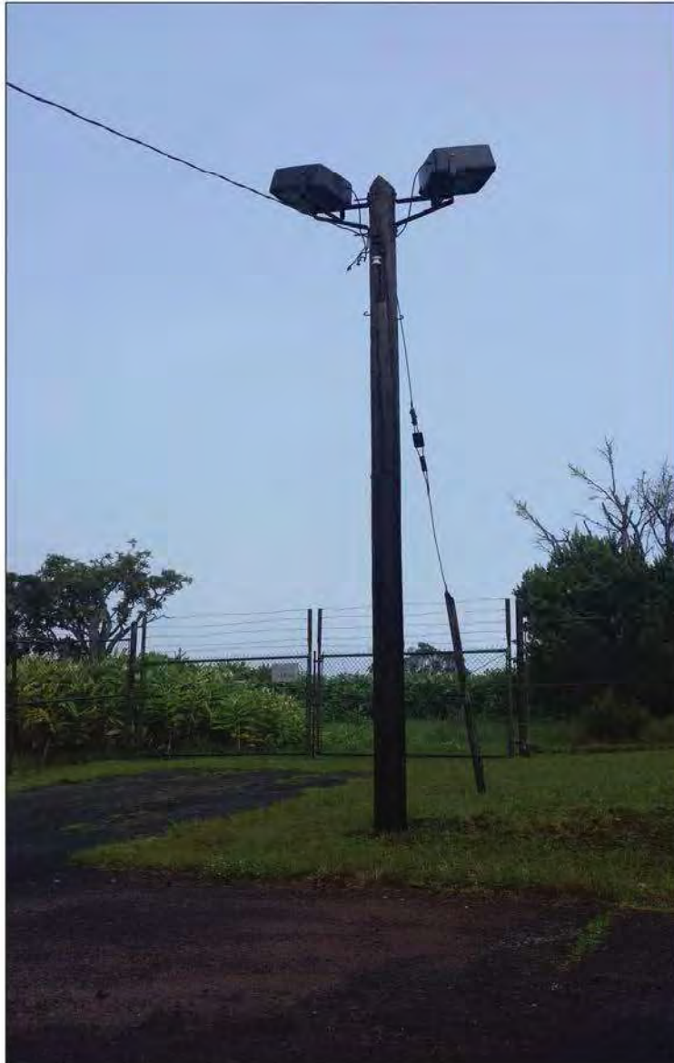
Perimeter Light_K: Two green bulbs, with full shielding, located in the most western corner of the installation.
