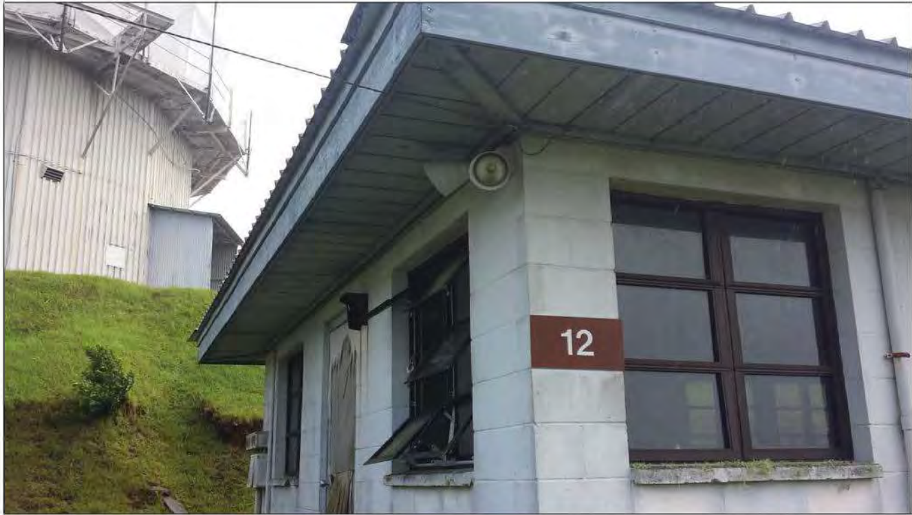
Building 12_Flood Light 1: Two white bulbs each with shielding and no motion detection (building appears to no longer be in use).
