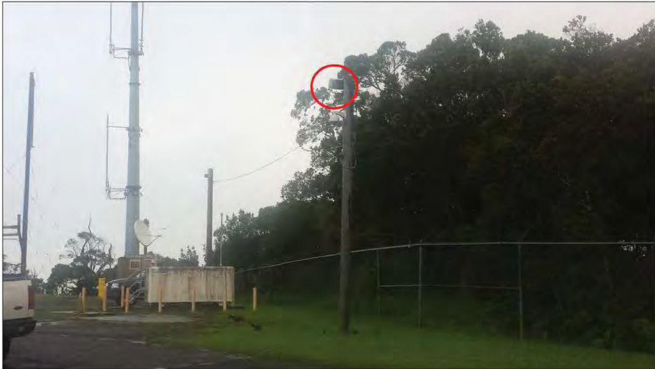
Perimeter Light_B: One green bulb, with full shielding, along the eastern fenceline.
