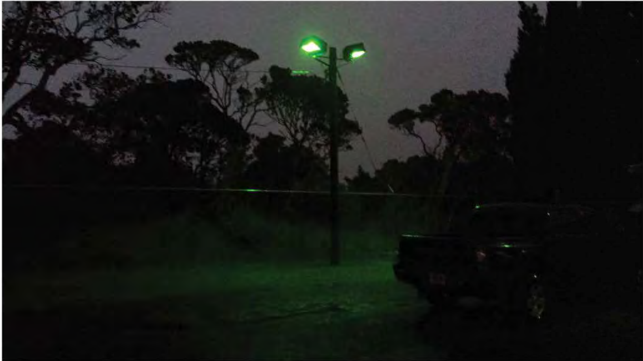
Perimeter Light_A: Two green bulbs, with full shielding (green lights on), northeast of guard shack.
