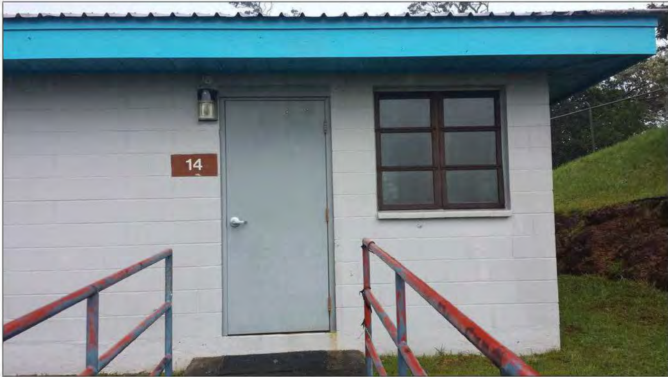
Building 14_Entryway Light 1: One white bulb with no shielding and no motion detection, southeast facing.
