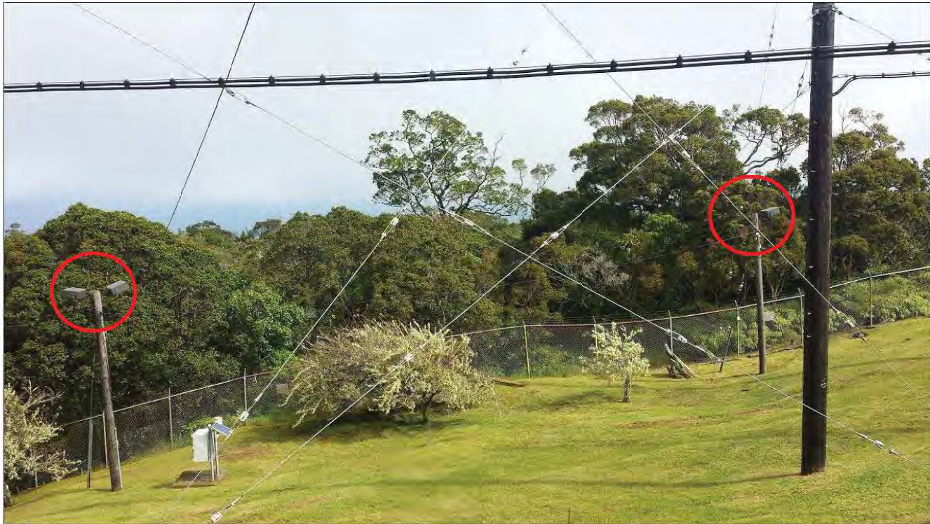
Perimeter Light_E : One green bulb, with full shielding (circle on the right)
