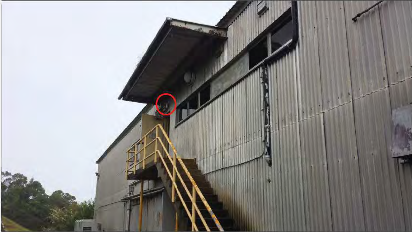
Building 1_Entryway Light 1: One white bulb, no shielding and no motion detection, 2 nd floor.
