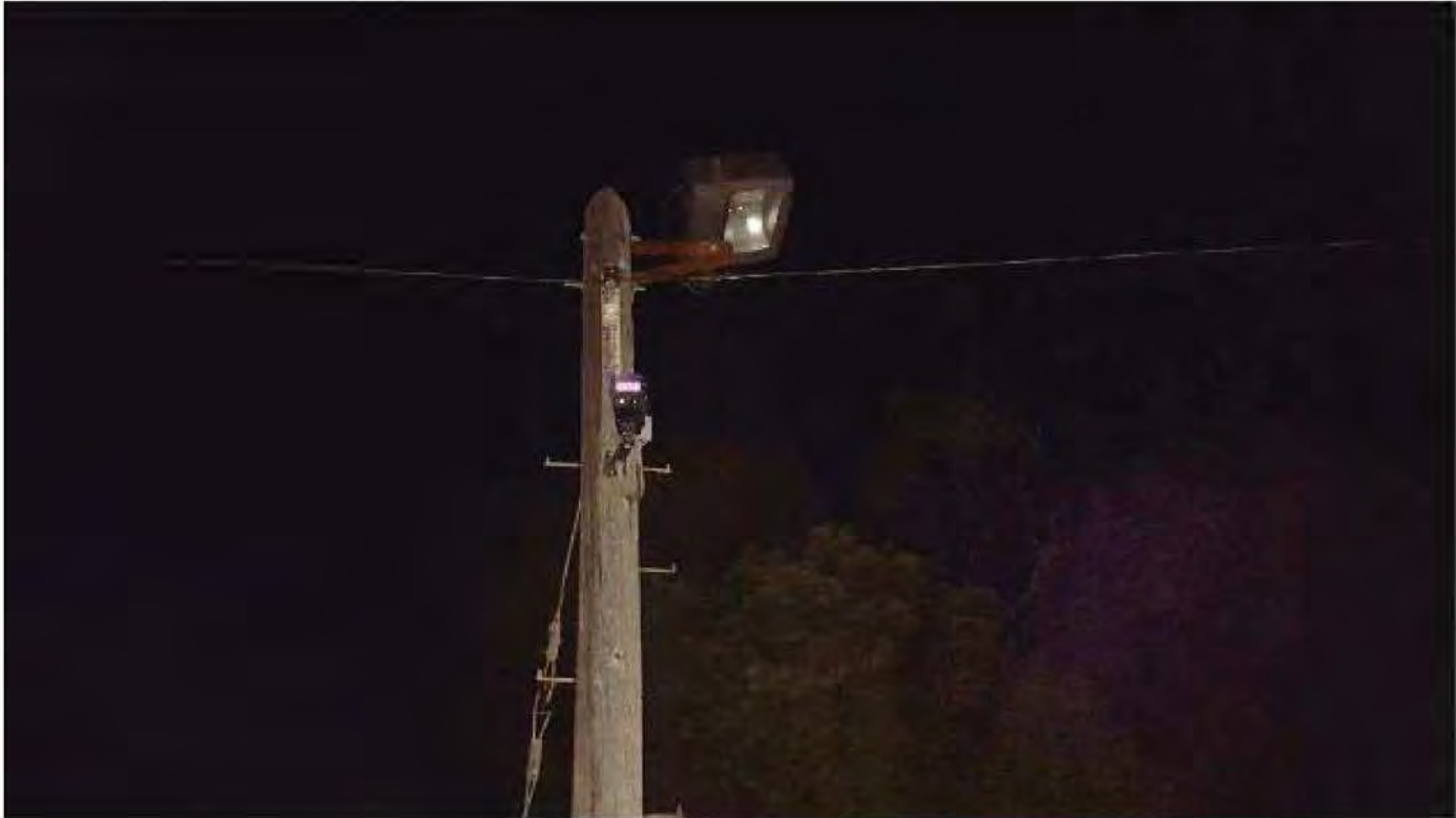
Perimeter Light_E (close up): One green bulb, with full shielding, light is currently not functioning.
