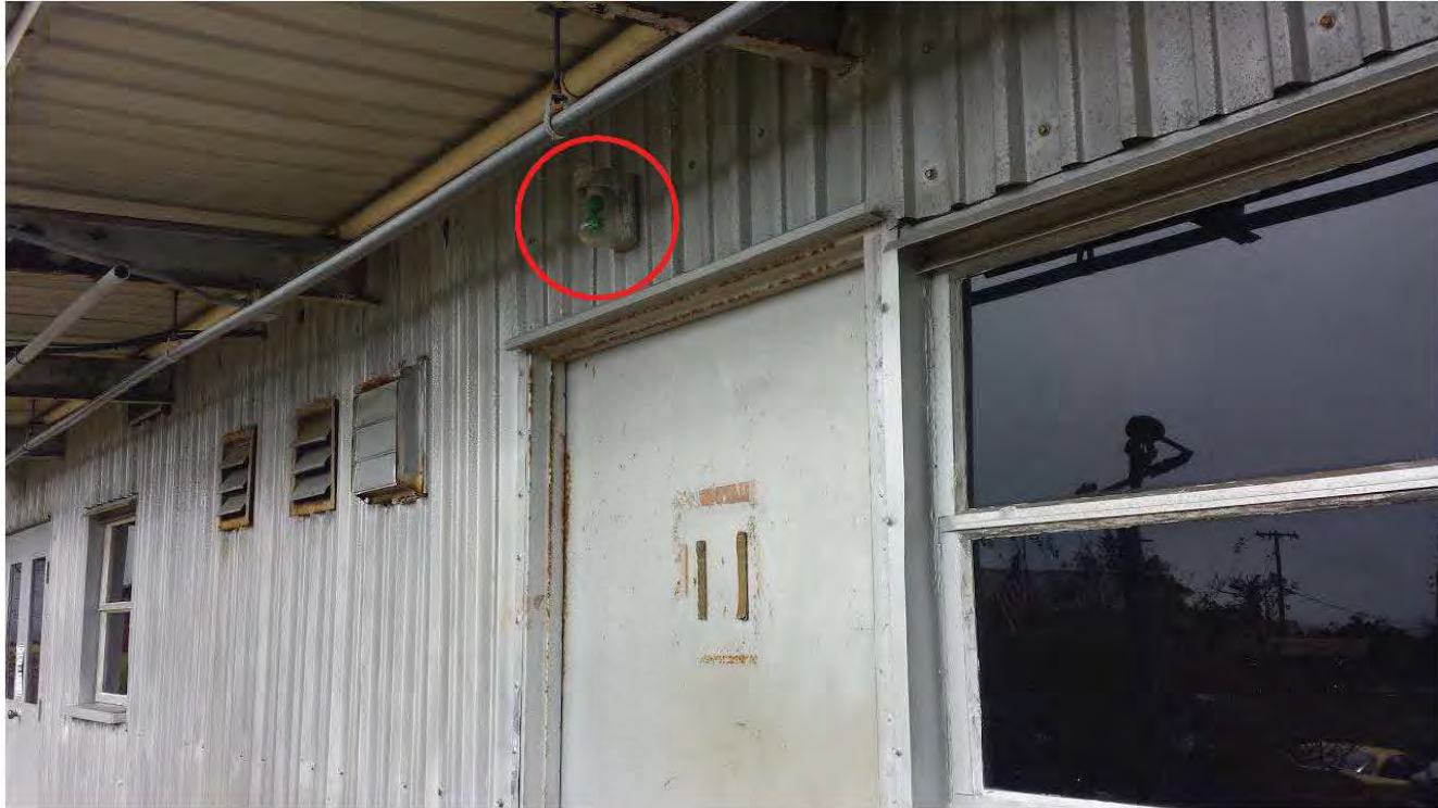
Building 1_Entryway Light 3: One green bulb with no shielding or motion detection, 1 st floor, southeast facing.
