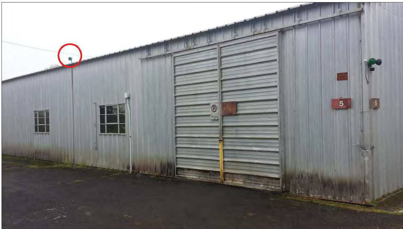
Building 5_Flood Light 4: One green bulb with no shielding and no motion detection, bulb is facing northeast and mounted onto of the top of the building.
