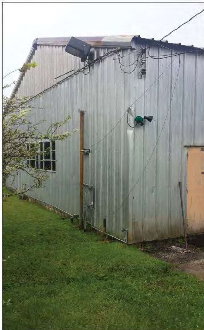
Building 5_Flood Light 3: Two green bulbs, both with shielding and motion detection.
