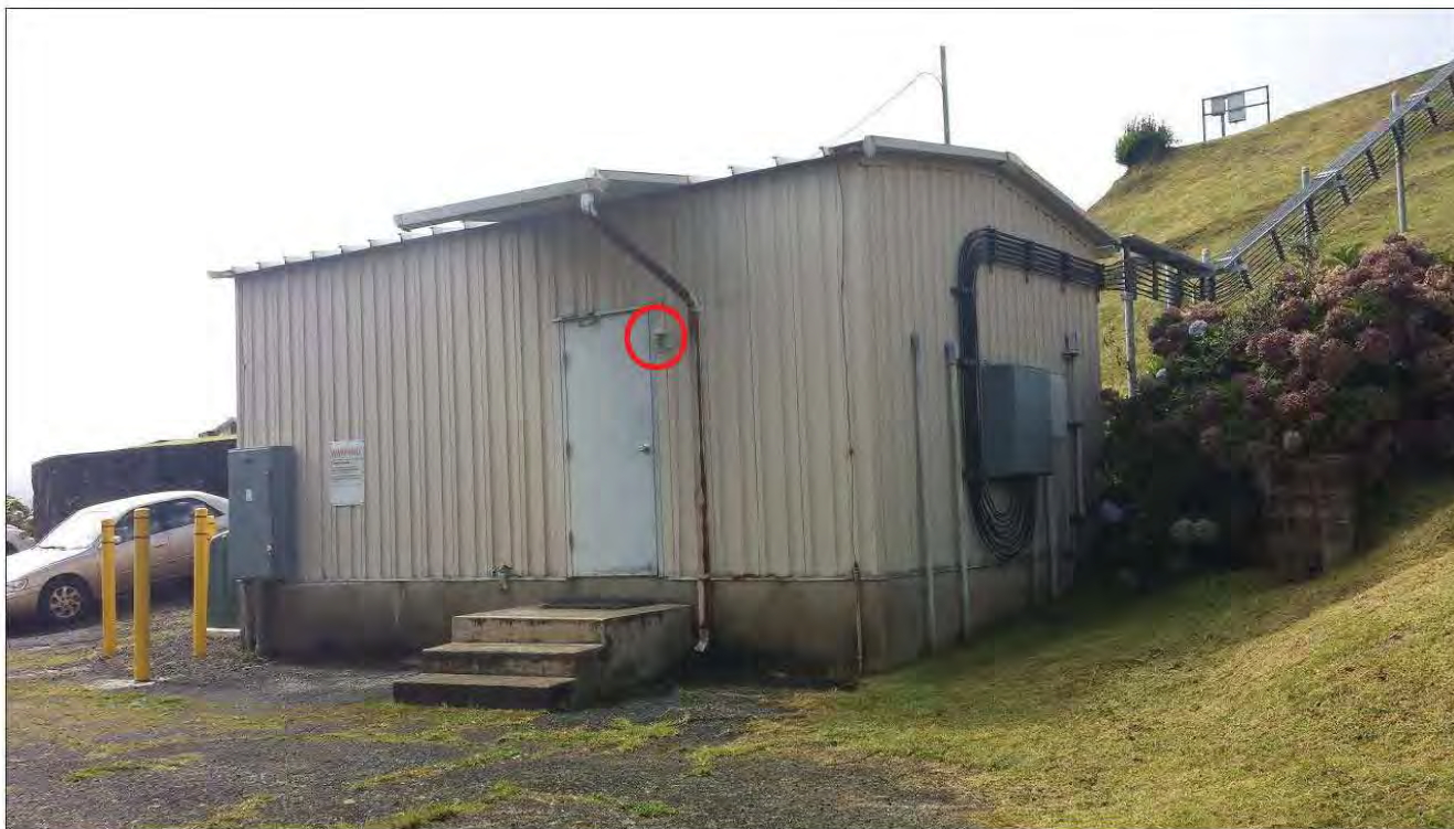
Power Shed (no building number)_Entryway Light 1: One green bulb with no shielding and no motion detection.
