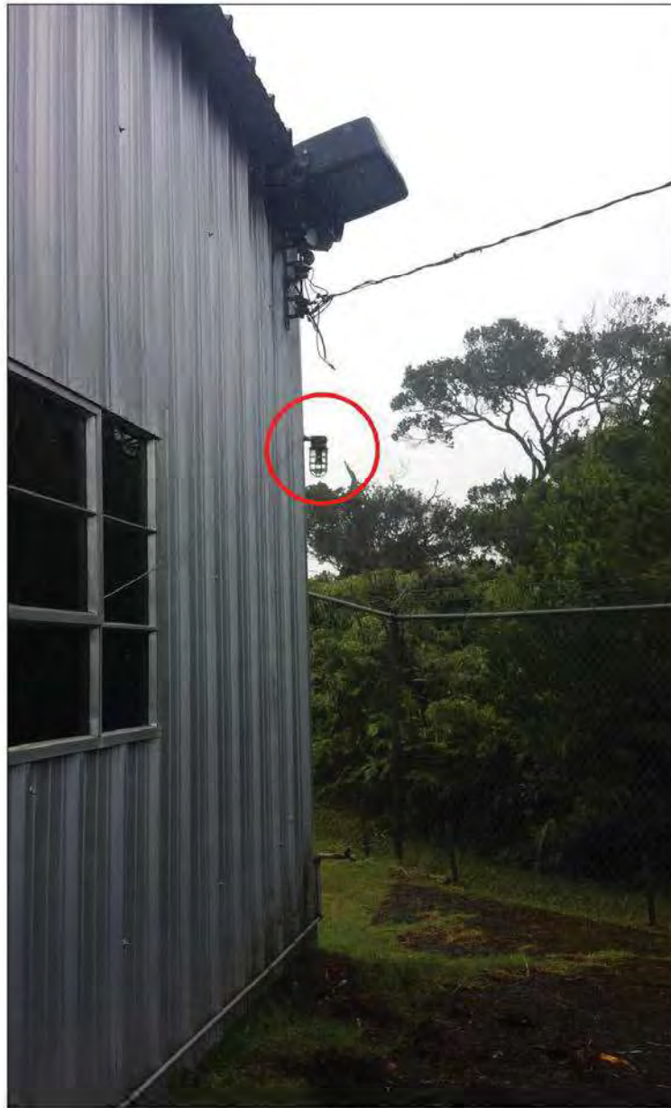
Building 5_Building Exterior Light 1: One green bulb with no shielding and no motion detection .
