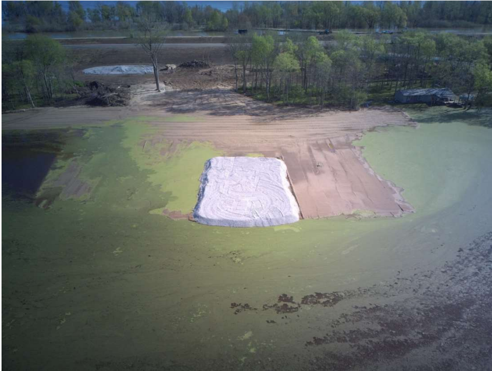
Figure 2. Remediated sand boil at the Black Hawk site. The gravel pad lies over the boil and extends into the borrow pit, surrounded on three sides by water.
