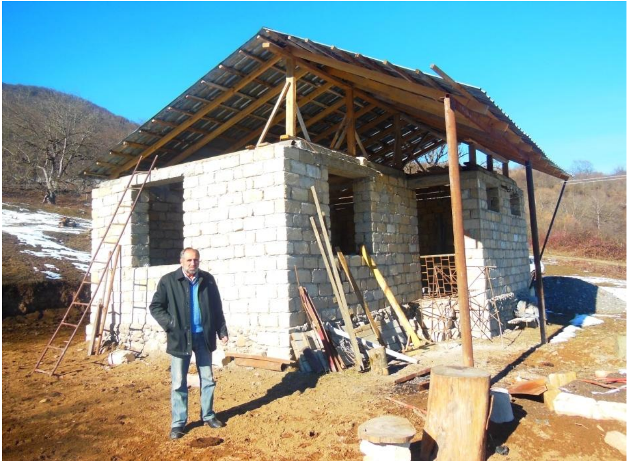
Above: the local Mayor Garik Sargisyan next to a new house being constructed on the cleared minefield funded by USAID
