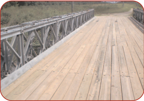
A 60 foot Double-Single Bailey was selected for this utility right-of-way access bridge near Orlando, Florida.
