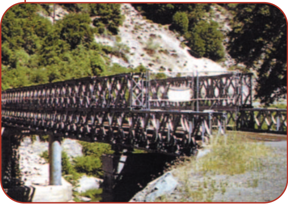
Pacific Gas & Electric Company, 215 ft. access bridge with 2 intermediate piers over the Feather River at Buck's Creek Powerhouse, California.
