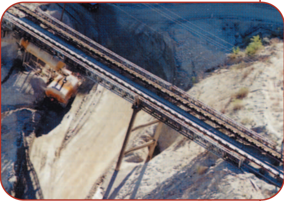
U.S. Army Corps of Engineers utilized a Bailey bridge system as a conveyor support for transporting over 19 million cubic yards of earth and rock for the construction of Seven Oaks Dam near San Bernardino, CA.
