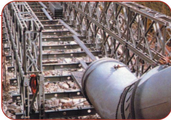
Montana Power Company, Mystic Power Plant, 160 ft. DDR Bailey carries 54" water pipe. Bridge components transported to site by helicopter.
