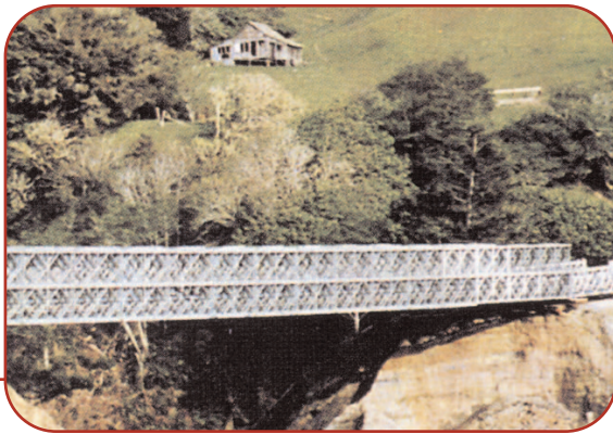
Clear span 200 ft. temporary TDR M2 Bailey bridge of California Hwy. 1. All components later reused in two 150 ft. temporary spans on Hwy. 395; now on standby, stockpiled for emergency or other use. California Department of Transportation.
