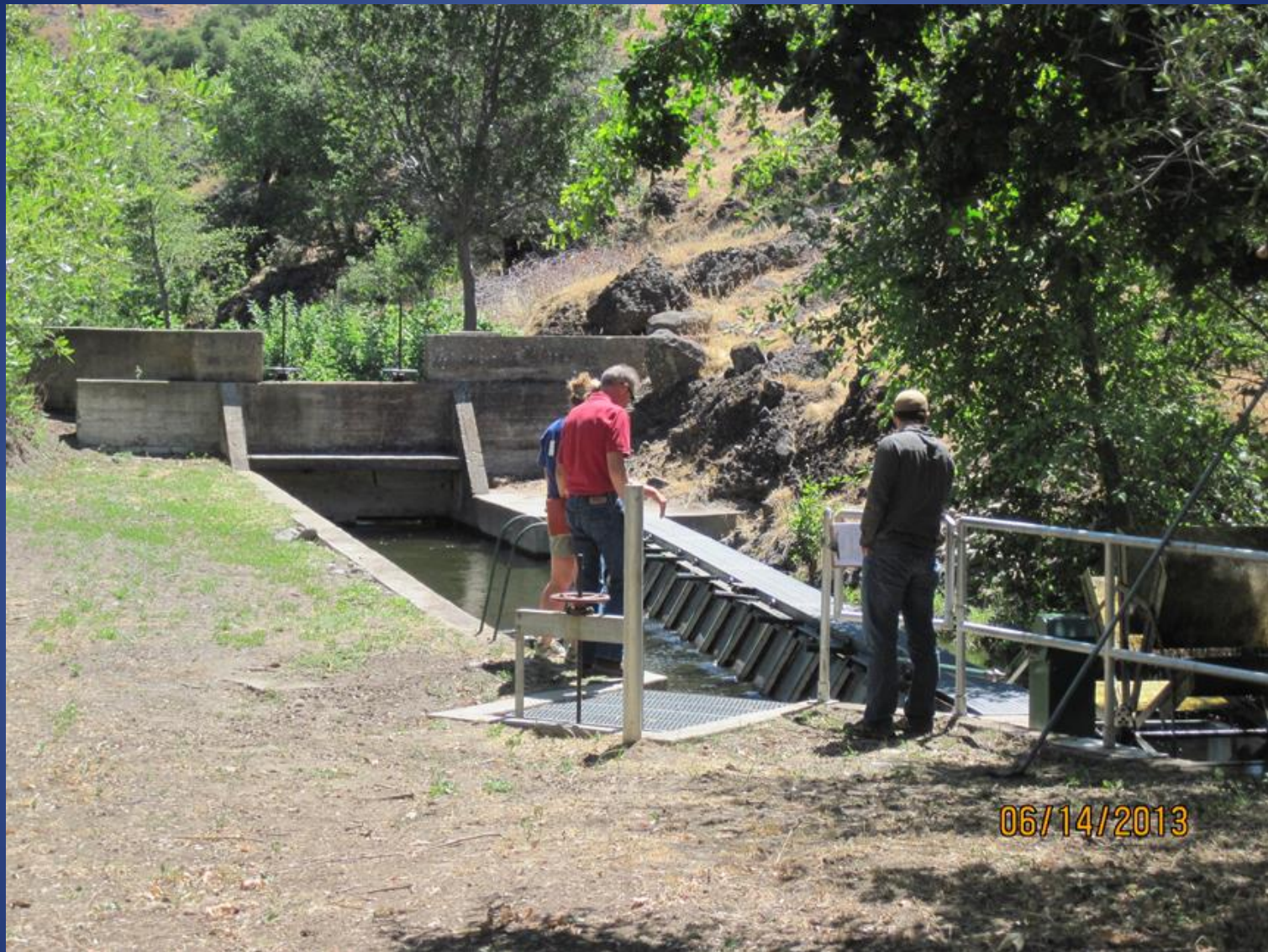
DCID screen and headgate
