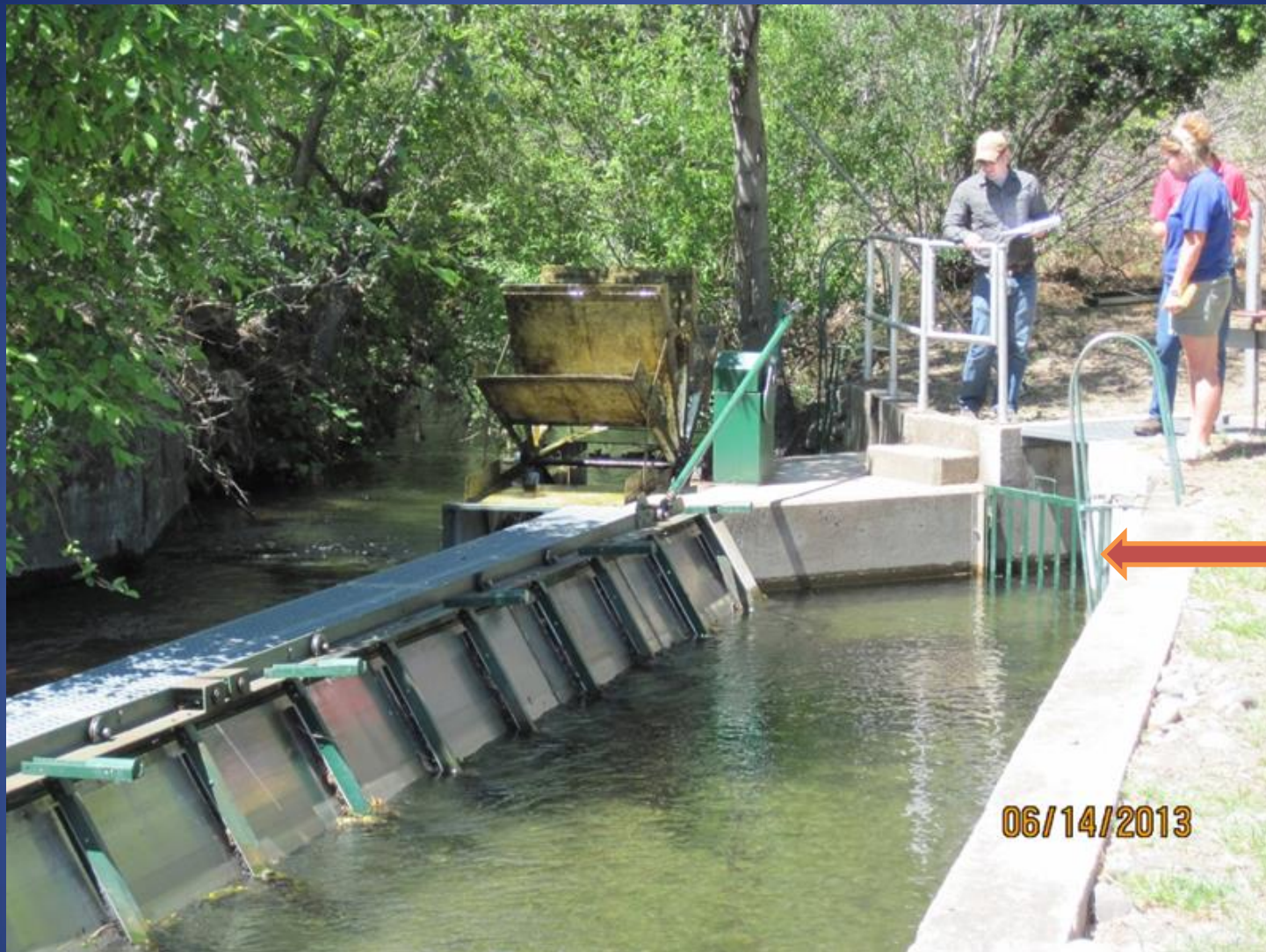
DCID screen and bypass entrance
