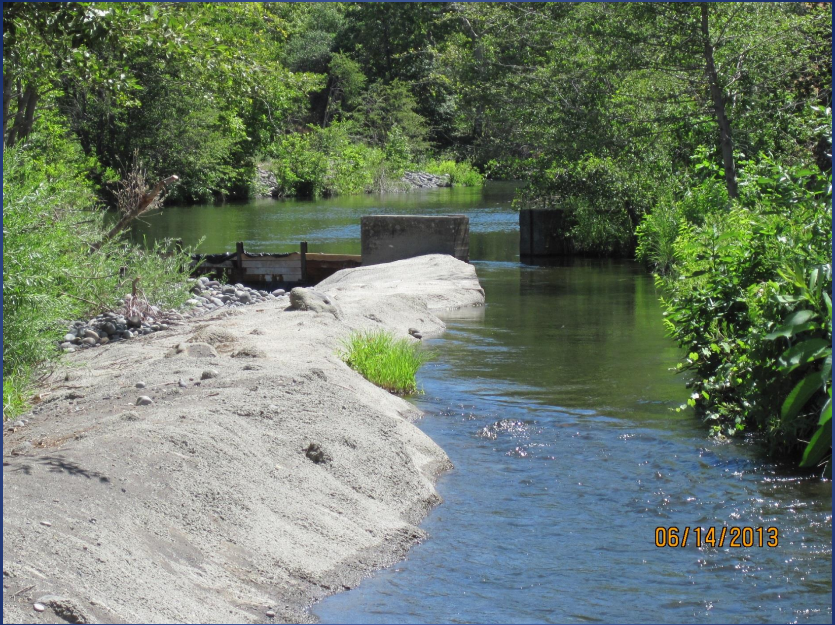
DCID ditch entrance and river left side of dam
