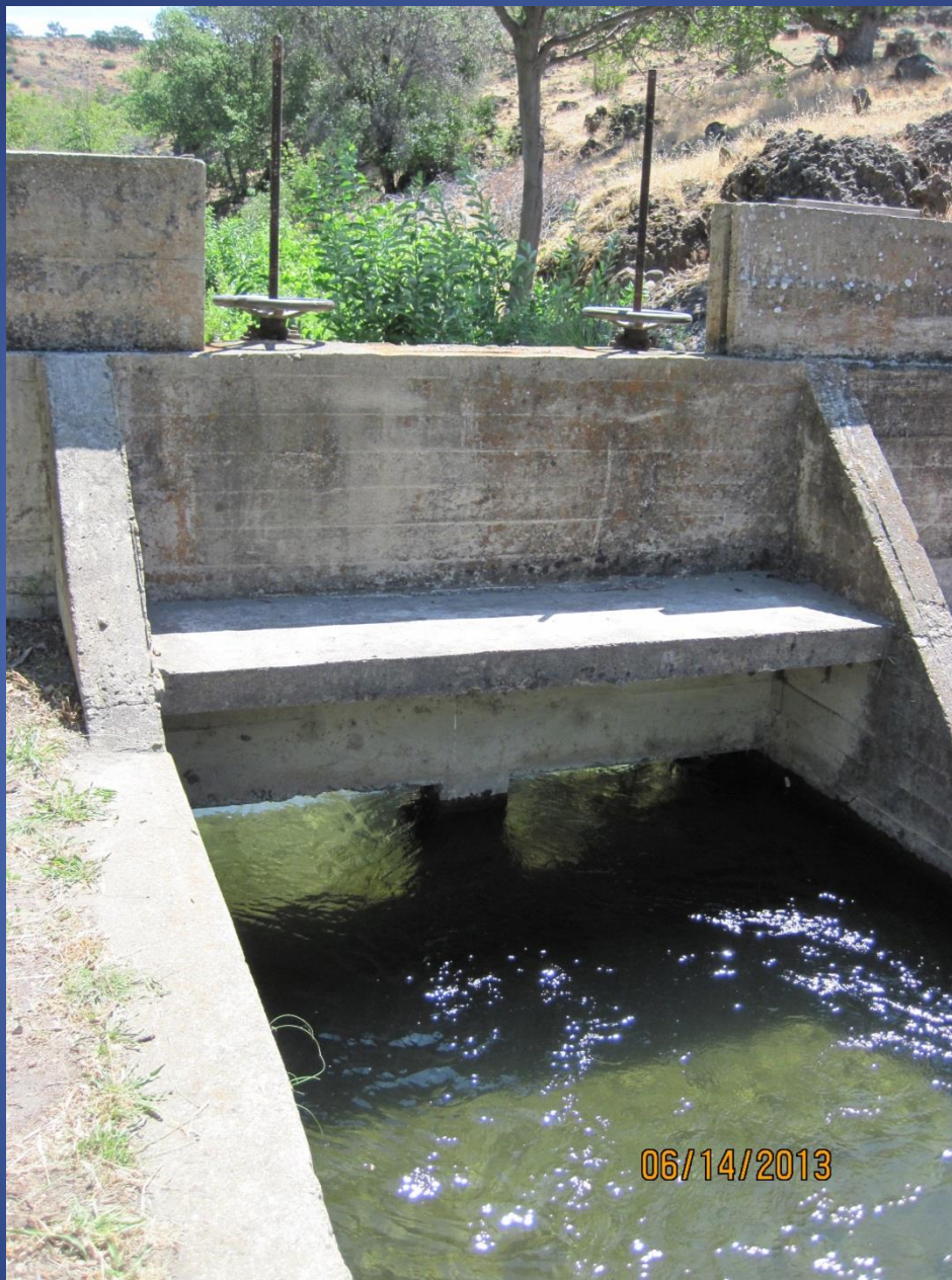
DCID headgate, downstream side
