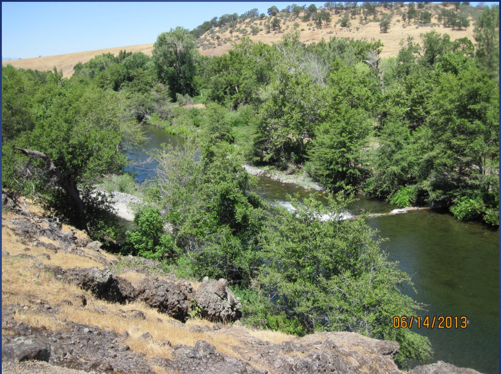
DCID dam from above, looking downstream
