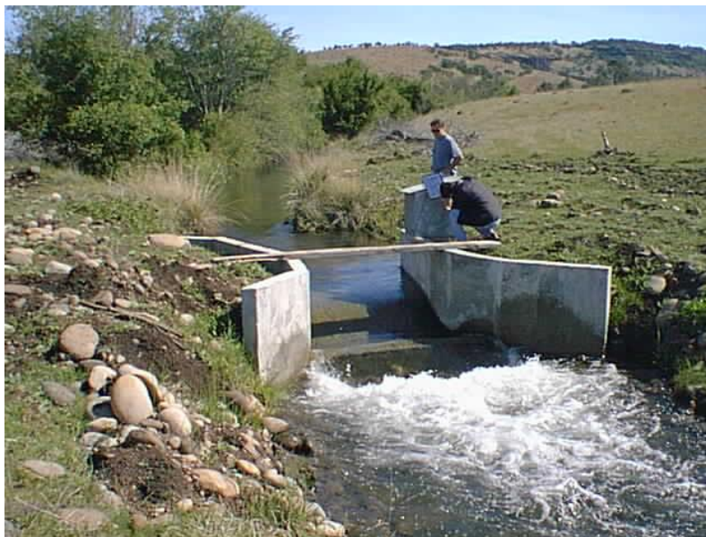
Figure 6. Parshall flume on Deer Creek (May 11, 1999). Photo: DWR
