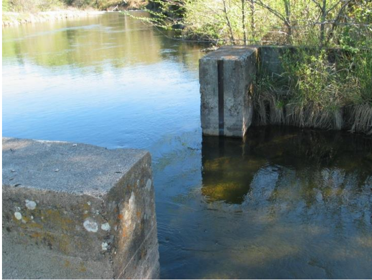
Figure 3. Diversion Ditch Weir Entrance (March 11, 2005). Photo: DWR
