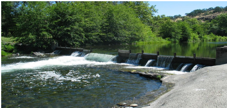
Figure 2. DCID dam without flashboards in the center section for fish passage (July 8, 2005, Deer Creek Flow = 135 cfs, DCID diverting 24 cfs). Photo: DWR
