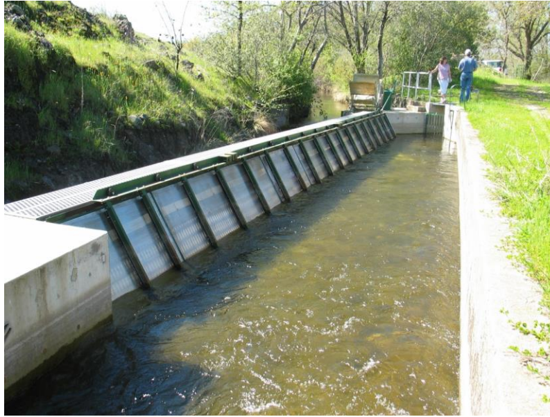
Figure 5. Fish screen structure (March 11, 2005). Photo: DWR
