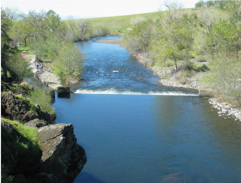
Figure 1. Deer Creek Irrigation Dam and Diversion (March 11, 2005). Photo: DWR
