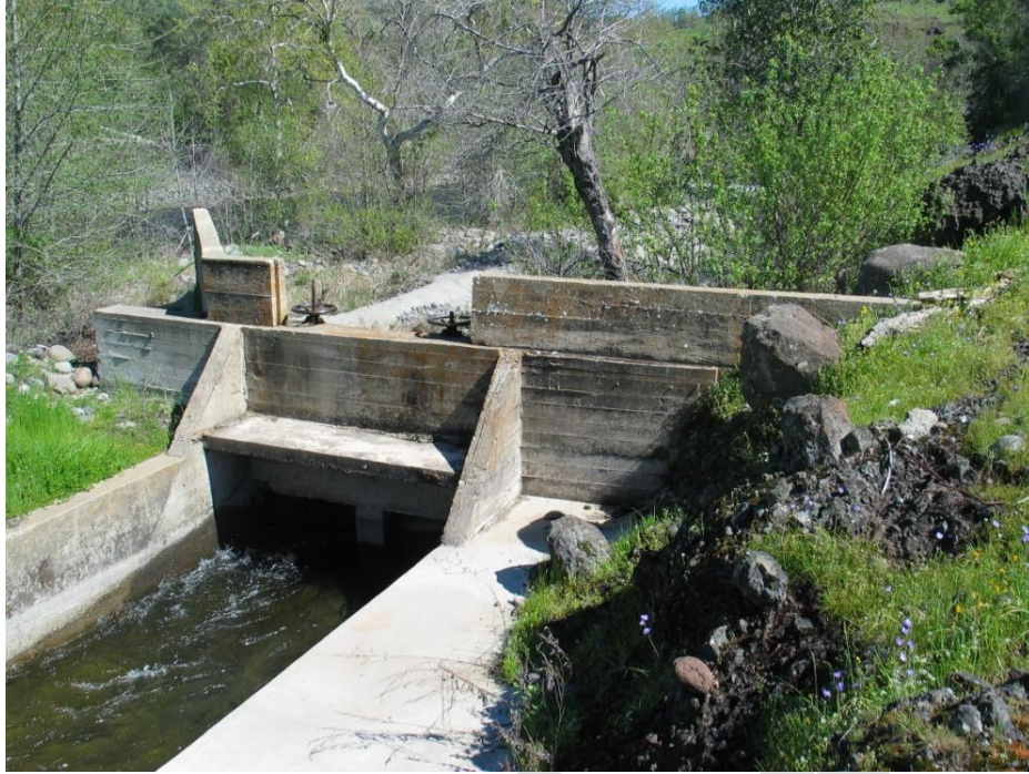
Figure 4. Headwall with two 48-inch vertical slide gates (March 11, 2005)
