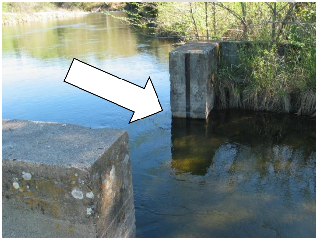
Figure 3. Diversion Ditch Weir Entrance (March 11, 2005)
