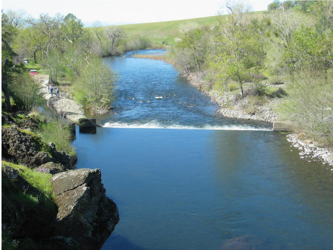
Figure 1. Deer Creek Irrigation Dam and Diversion (March 11, 2005)
