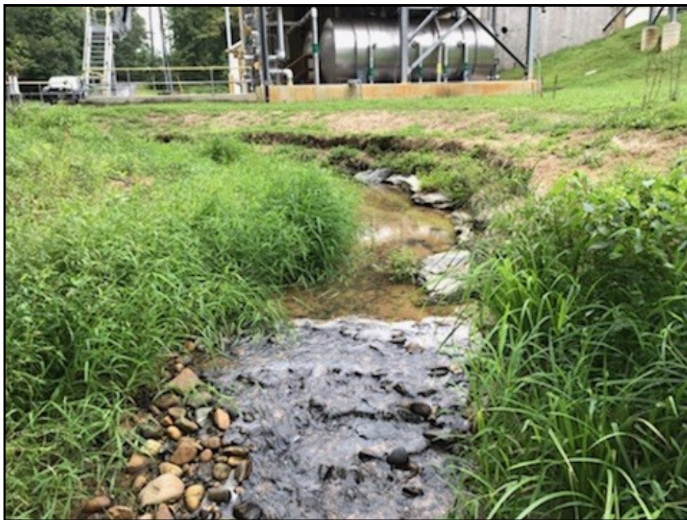
Photo 12. Third Quarter monitoring (9/10/2018) facing upstream near Cross Section 2.
