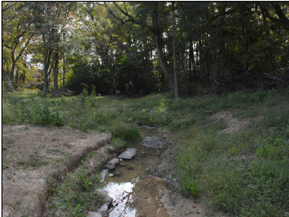
Photo 2. Typical condition of site facing downstream from middle of site. Soil lifts, stone toe, grading, and vegetation are performing as designed.
