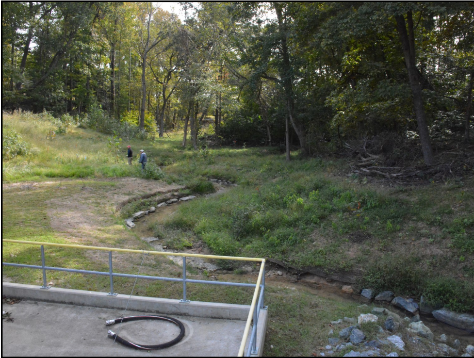
Photo 1. Typical condition of site facing downstream.
