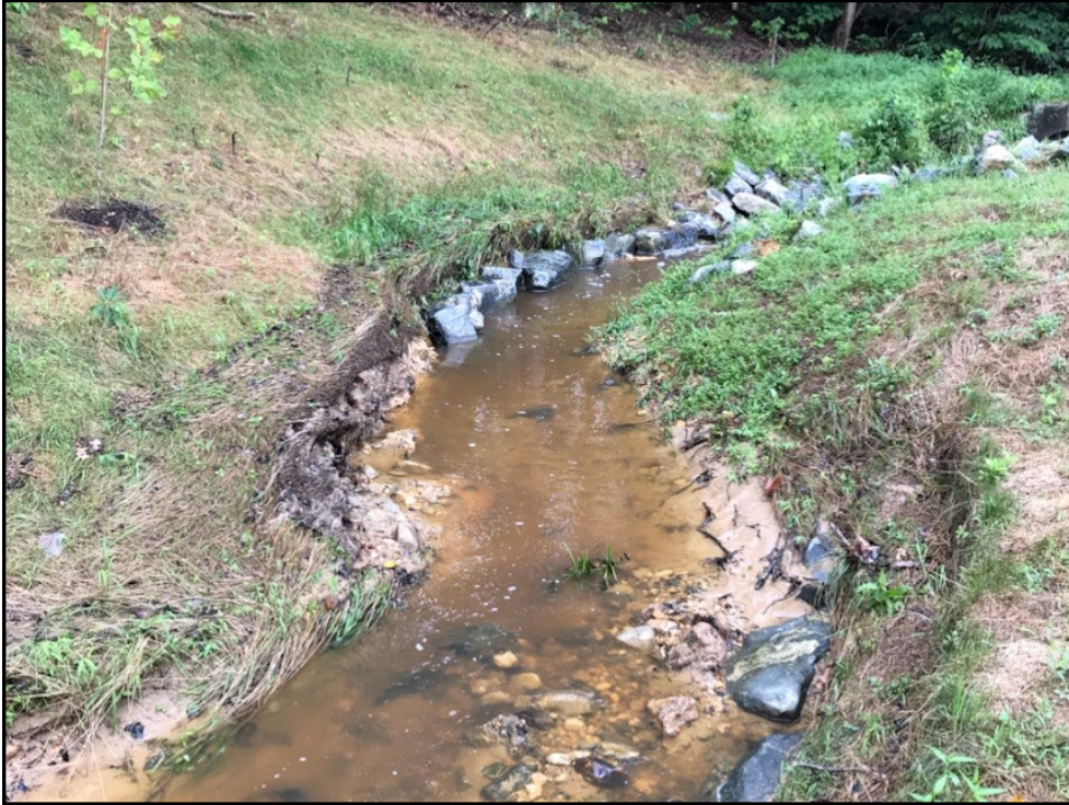
Photo 9. Post-storm inspection on 7/23/2018 following 5.41-inch storm (facing upstream). Slight bank scour at end of stone toe.
