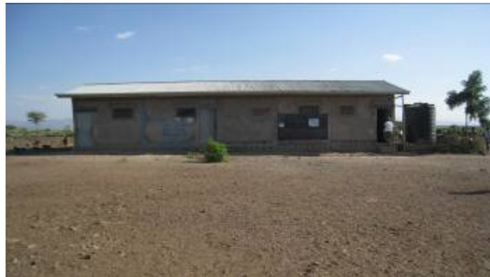
Photo 19 (left). School latrine facility - Legadini. Photo 20 (top right). Rainwater harvesting water supply - Legadini Photo 21. (bottom right). School at Legadini.
