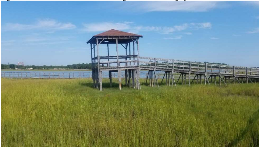
Figure 5: Nature Trail Platform sinking into JBLE-Langley Marsh
