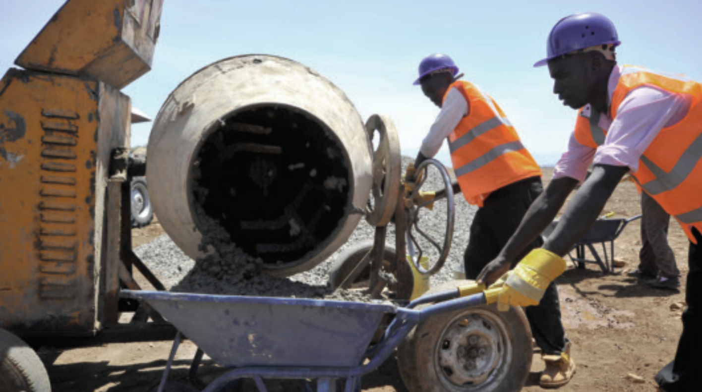
Construction workers prepare the new biomass energy power plant in Marigat, Kenya, as part of a USAID-fostered partnership between Cummins Cogeneration Kenya Ltd. and the Kenyan Government. Improving the host government's ability to evaluate and select the most effective investments can have a huge impact on economic growth. PHOTO: USAID
