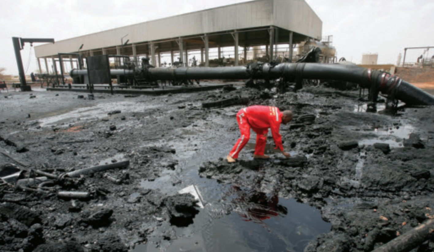
A Sudanese worker inspects damage to a burnt oil-processing facility in Heglig, Sudan. African countries hold vast mineral and energy wealth that could be converted into economic infrastructure, social progress and human capital. PHOTO: ASHRAF SHAZLY / AFP
