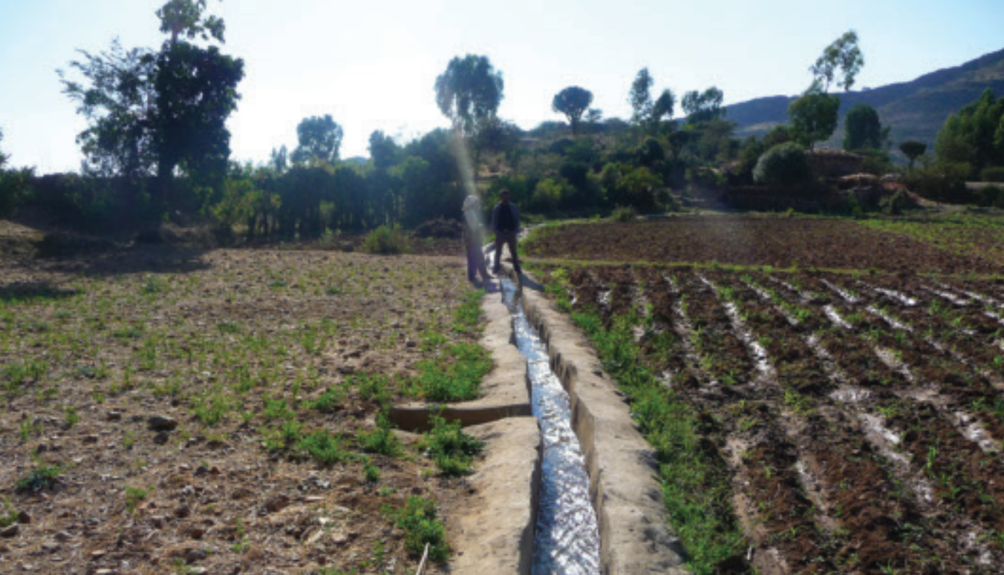
Technological solutions have the ability to catalyze financing for resilience dividends. Crop and climate modeling led to the financing of this irrigation site at Awda-Guanda watershed in Ethiopia. Irrigation canals such as this one are built by communities in exchange for crop insurance or food aid.
