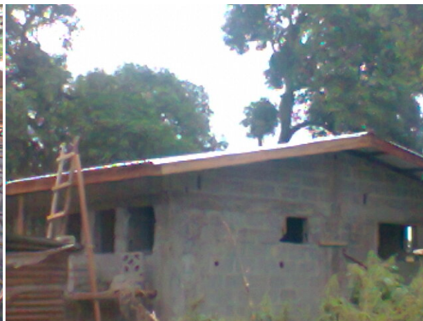
Latrine with roof installed
