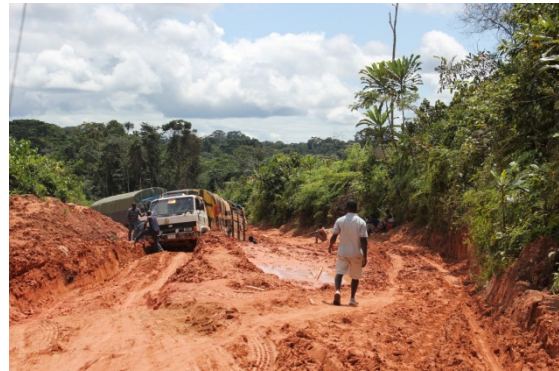
Difficult Road Conditions: The Main Road Between Bong and Nimba counties
