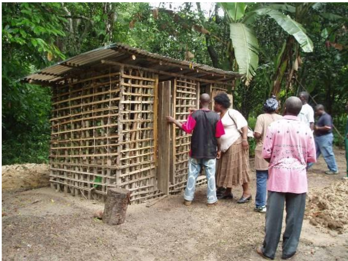
Fig 3 - Latrine under construction, Gparbolu
